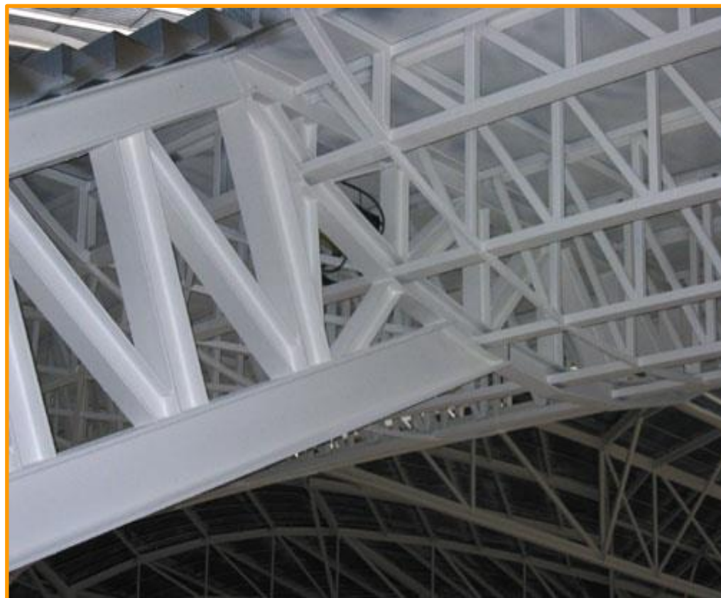
Columns protected with industrial intumescent coating and top coated with fireproof coating
